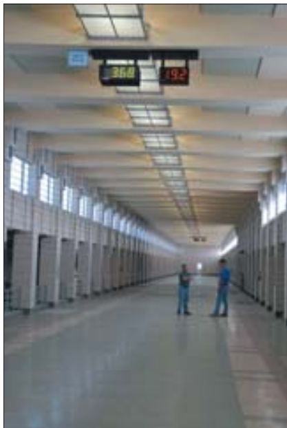
Operating gallery in the GCWW filter building.
